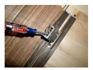
Step 5: Remove the cords from the cord lock. You can now unscrew the cord lock and replace it in exactly the same position. Note that the angled side of the cord lock is towards the end of the head rail.
